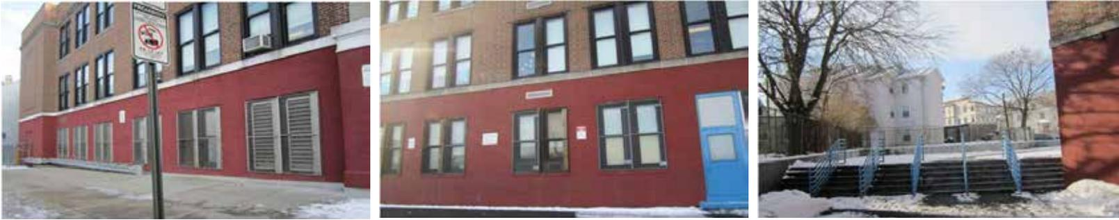
The site is Paterson School #8 located at 45 Chadwick Street. There is little to no identifiable slope to the site. There are no external downspouts on the building. The pavement appears to be in good condition, and the site is almost entirely impervious. Depaving and stormwater planters could be used to reduce runoff.
